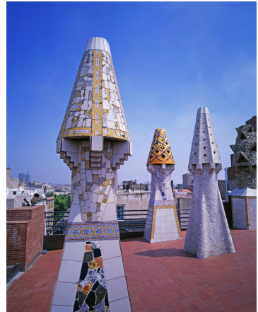
(2) Palau Güell rooftop, Barcelona, 1886 - 1890
